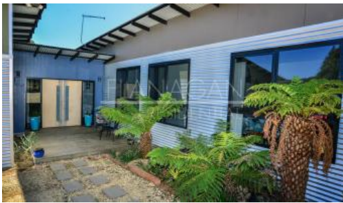
44a New Ecclestone Road St, Riverside
