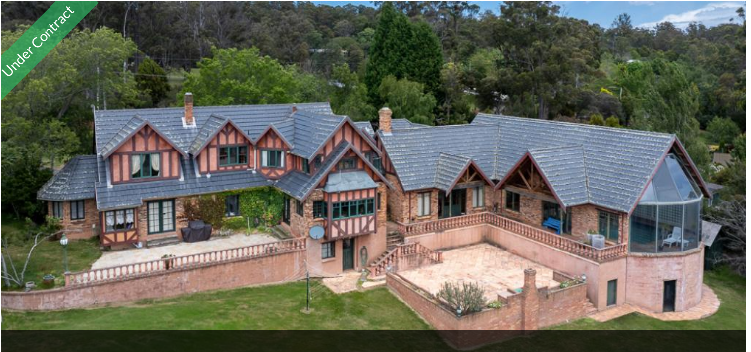
72 New Ecclestone Road, Riverside
